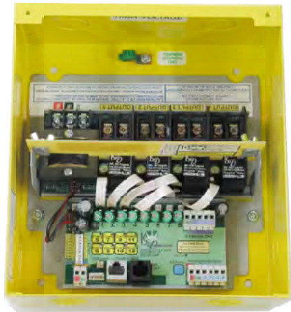
GR 2404 iDim or DH with no Emergency loads.
