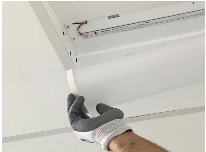
D. Press Lens and Trim Ring together into other End Plate and align pins to keyholes on the end plate.
